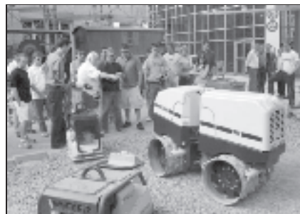
Student operating a remote controlled compactor at a museum of safety
