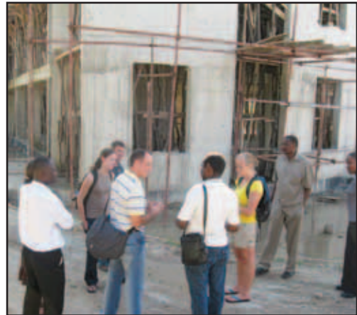
New building for University of Dar es Salaam's Business School
