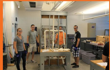
Students in BCN 4510 Mechanical Systems dry fit a drain, waste, and vent system for a bathroom.
